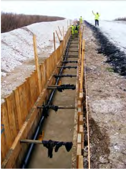
Figure 41 – Cable installation in an open cut trench
