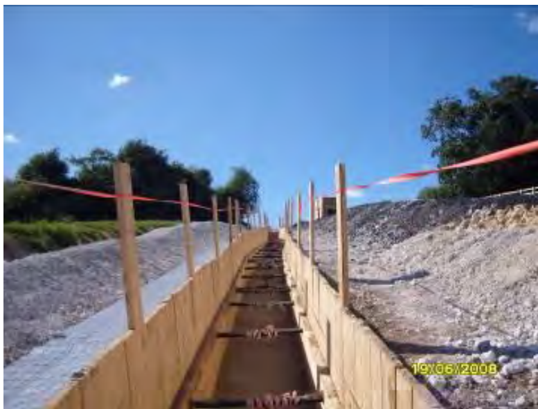
Figure 37 – A close-timbered cable trench
