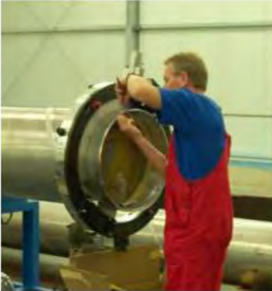
Figure 61 – GIL weld edge preparation prior to connection
