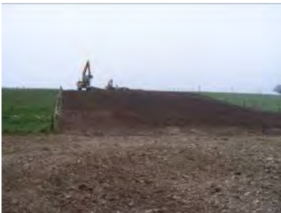
Figure 44 – Topsoil replacement
