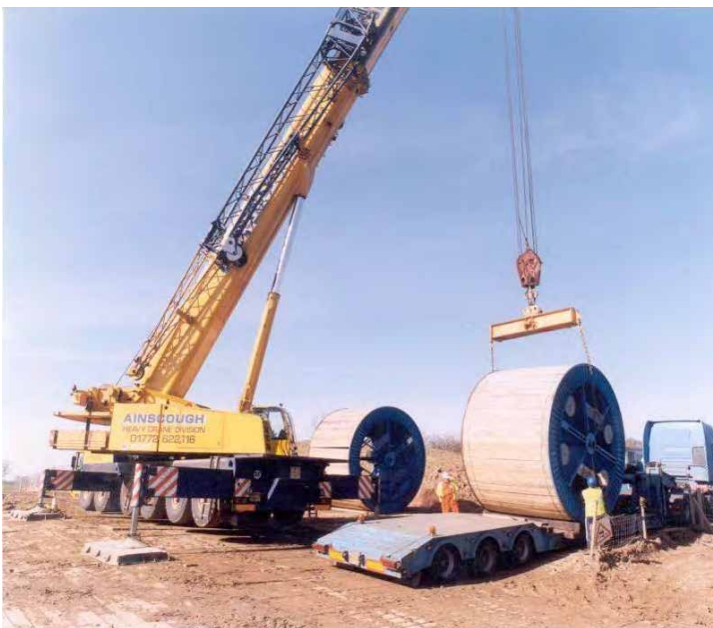
Figure 40 – Offloading cable drums
