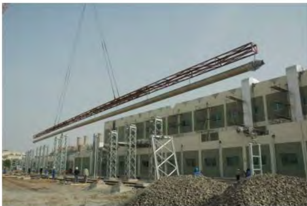
Figure 62 – GIL segment being lifted into position
