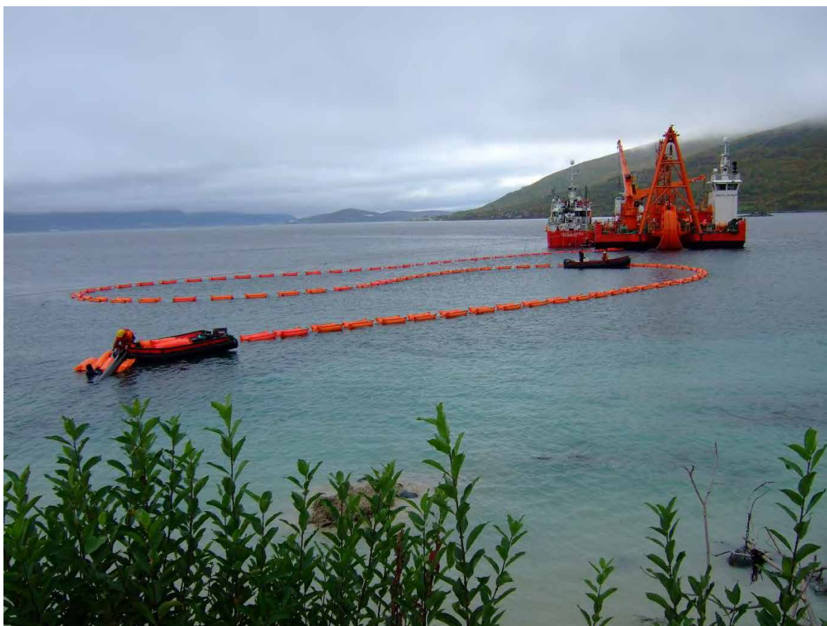
Figure 55 – Cable laying vessel shore landing installation
