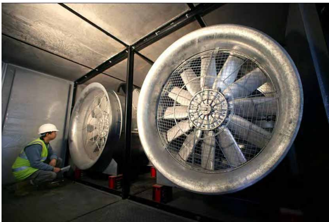
Figure 46 – Air cooling fans during installation
