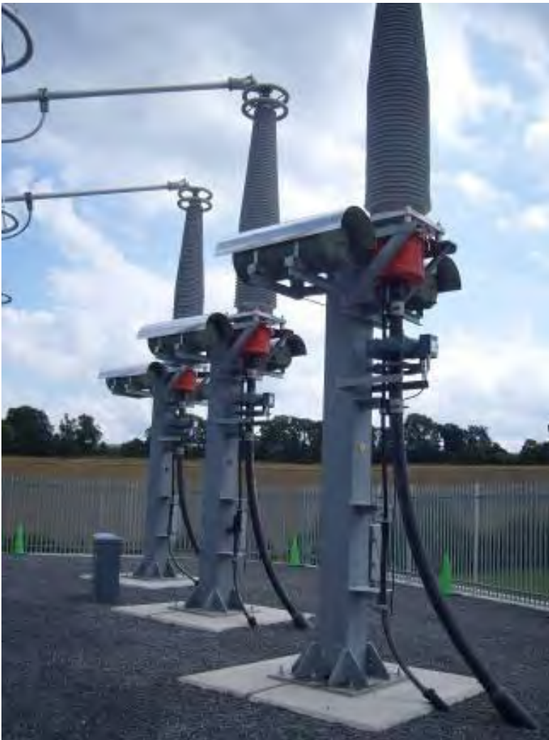
Figure 22 – 400kV terminations installed near Goring
