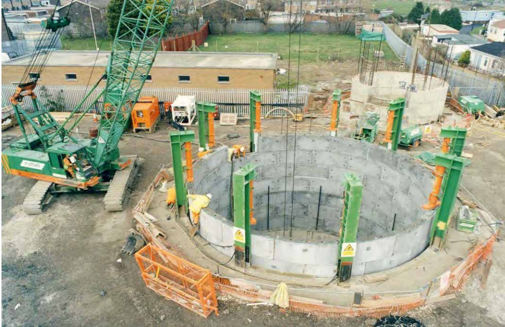
Figure 67 – Hydraulic jacks on caisson technique shaft construction
