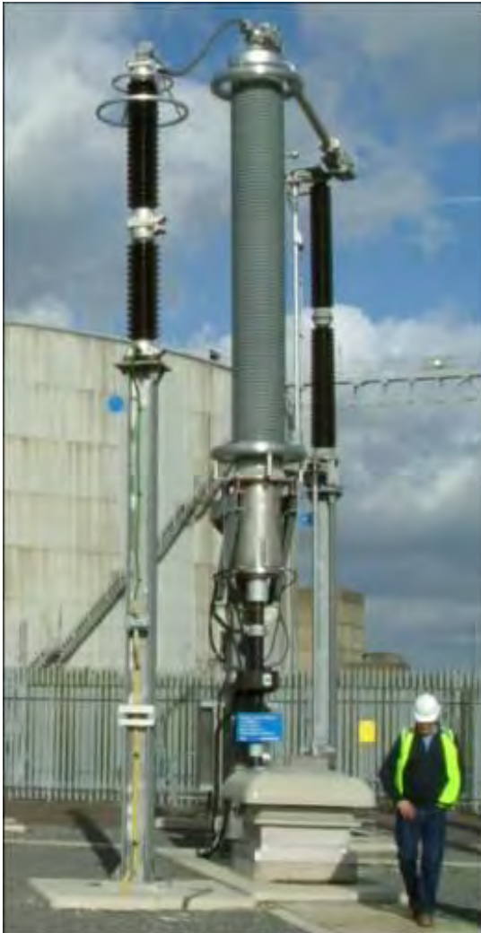
Figure 21 – 400kV cable outdoor sealing end (ODSE) termination
