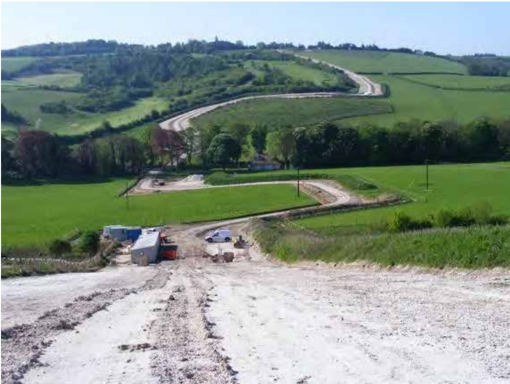
Figure 35 – 400kV cable swathe at the Goring Gap
