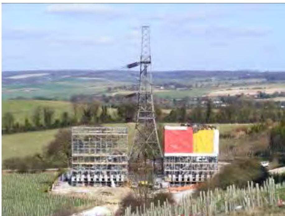
Figure 23 – Weatherproof enclosure for cable termination assembly
